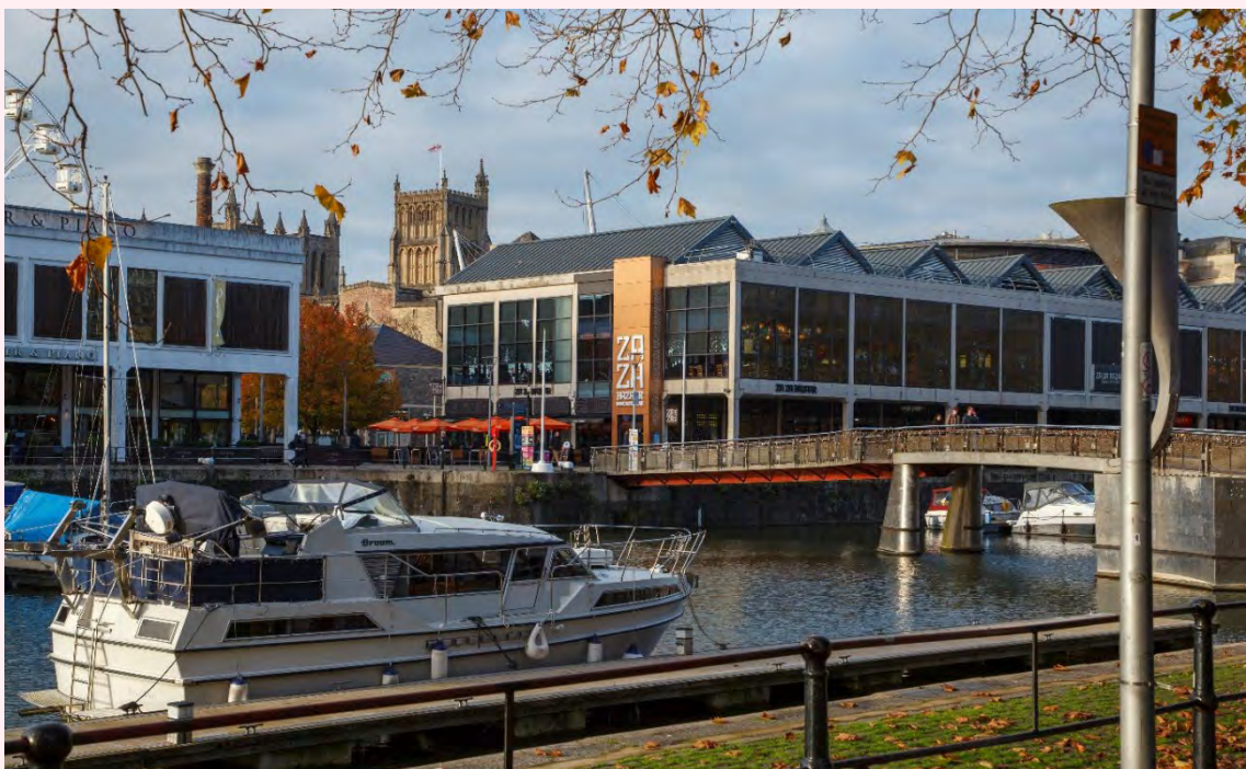
Above: The view from Narrow Quay illustrating the architectural and visual prominence of the Cathedral in dockside views. V-shed on 1926 is on the left, with U-Shed on the right. The visual effect of the saw-tooth roof profile adds skyline interest. 39 degree field of view from Narrow Quay
